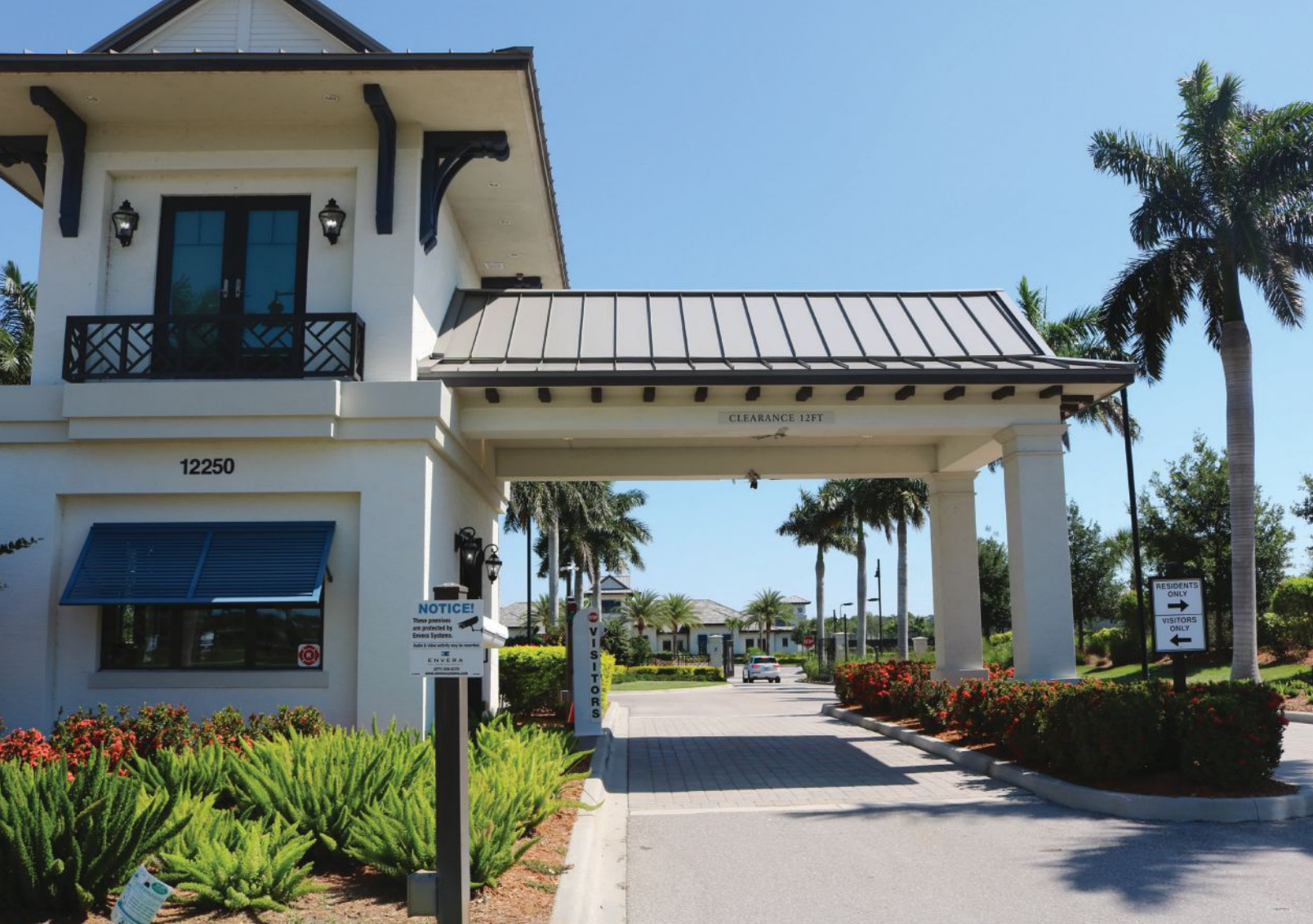
Photos courtesy of Envera Systems
